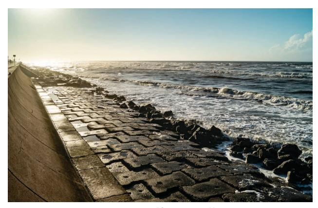
Figure 46. Curved face retaining dike
